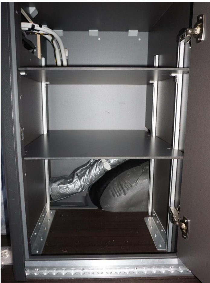
Figure 8. Positioning of aluminium tracks and shelves
