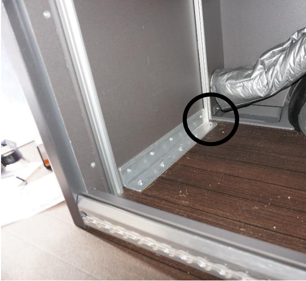
Figure 6. Positioning of aluminium track (B) left hand side.
