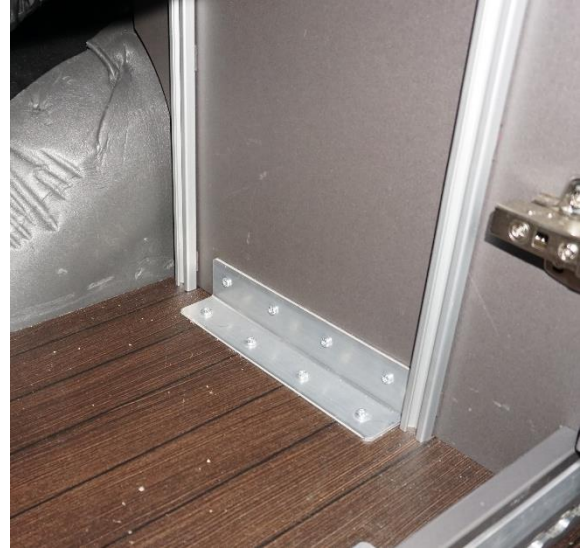
Figure 7. Positioning of aluminium track (B) right hand side.
